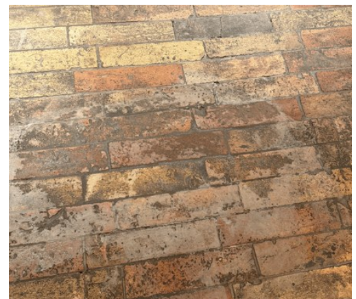
Kitchen flooring and finish details
